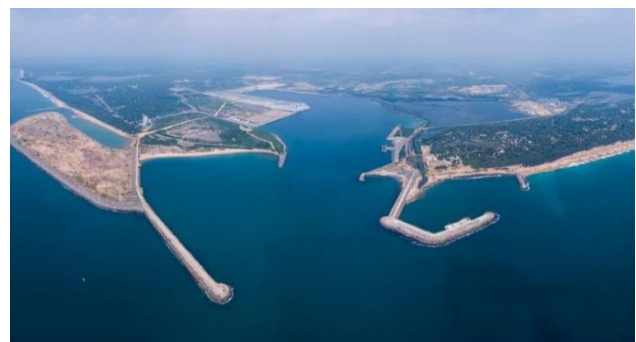
Figure 5. Breakwater of Hambantota harbour
