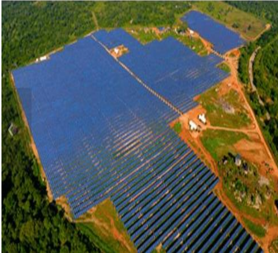
Figure 4.2: Welikanda Solar Power station.
