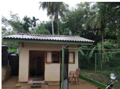
Figure 4. BWRO Facility building
