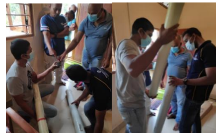
Figure 5. Inserting the new BWRO membrane into the pressure vessel
