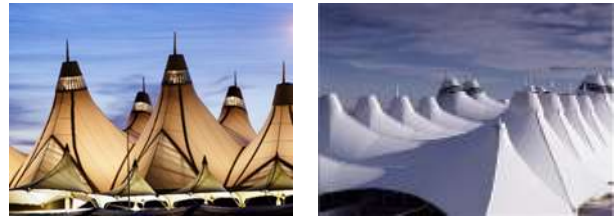
Figure 5: Roof structure of the Denver International Airport
