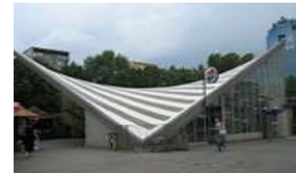
Figure 10: Roof of the Warszawa Ochota railway station, Warsaw Poland
